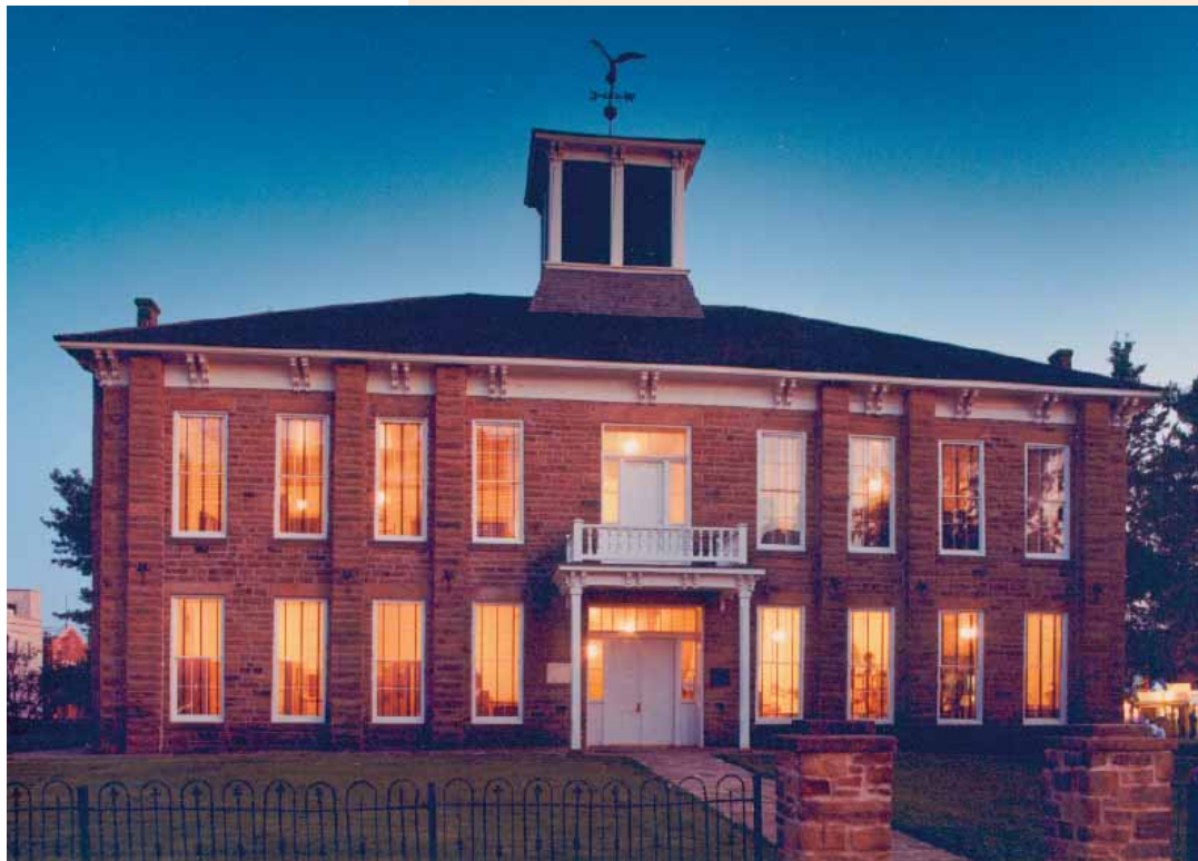
CREEK COUNCIL HOUSE MUSEUM
